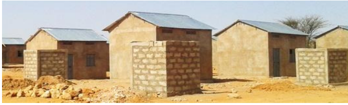
Construction of permanent shelters in Gaalkacyo, Mudug. Photo: Mohamed Abdulkadir/DRC
