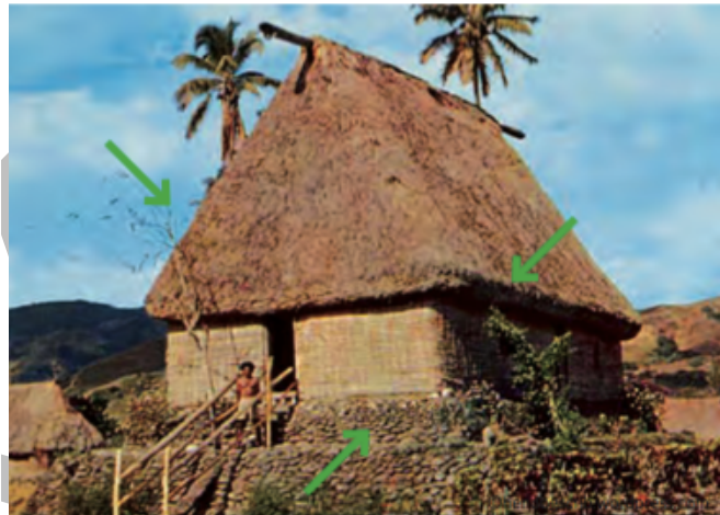
Elevated stone platform for protection from floods and soil erosion. Small eaves and steep roof for reduced vulnerability and improved durability
