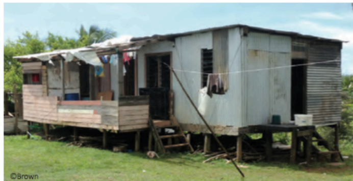
Transitional CI sheet housing: elevation on stilts for better protection from floods
