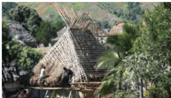
A net of woven reeds is applied on the rafters to better fix the thatching
