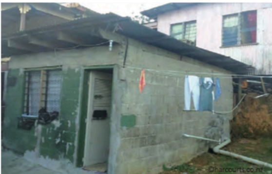
Formal low-cost housing: cement block masonry with anchoring for roof structure
