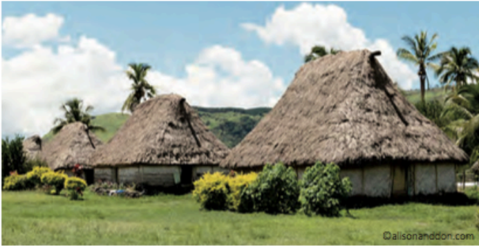
Traditional housing: lightweight flexible construction and 4-slope hipped roof for better wind resistance
