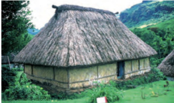
Traditional house: woven mat walls are fixed on the outside with additional wood elements to improve resistance to wind pressure; the top of the roof is reinforced with an additional layer of special grass tied to a timber beam protruding from two sides of the roof
