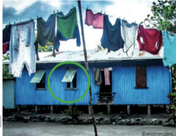
CI sheet house: tilting shutters can be easily fixed during cyclones
