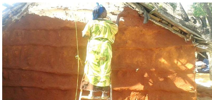
Renovation of shelters in Kismaayo Photo: Abdirahman Farah /ARC
