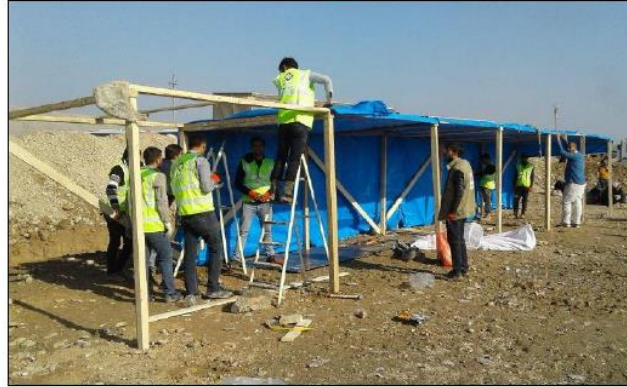
Picture from PiN on the use of BESKs as shading at Bartella screening site
