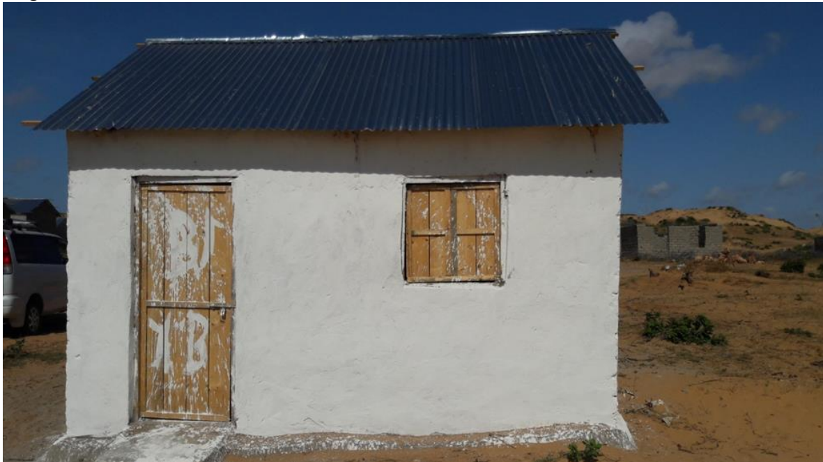
Front View of a completed WRRS Adobe block shelter 1
