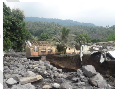
Figure 1 Damage to Waluweibue Village
