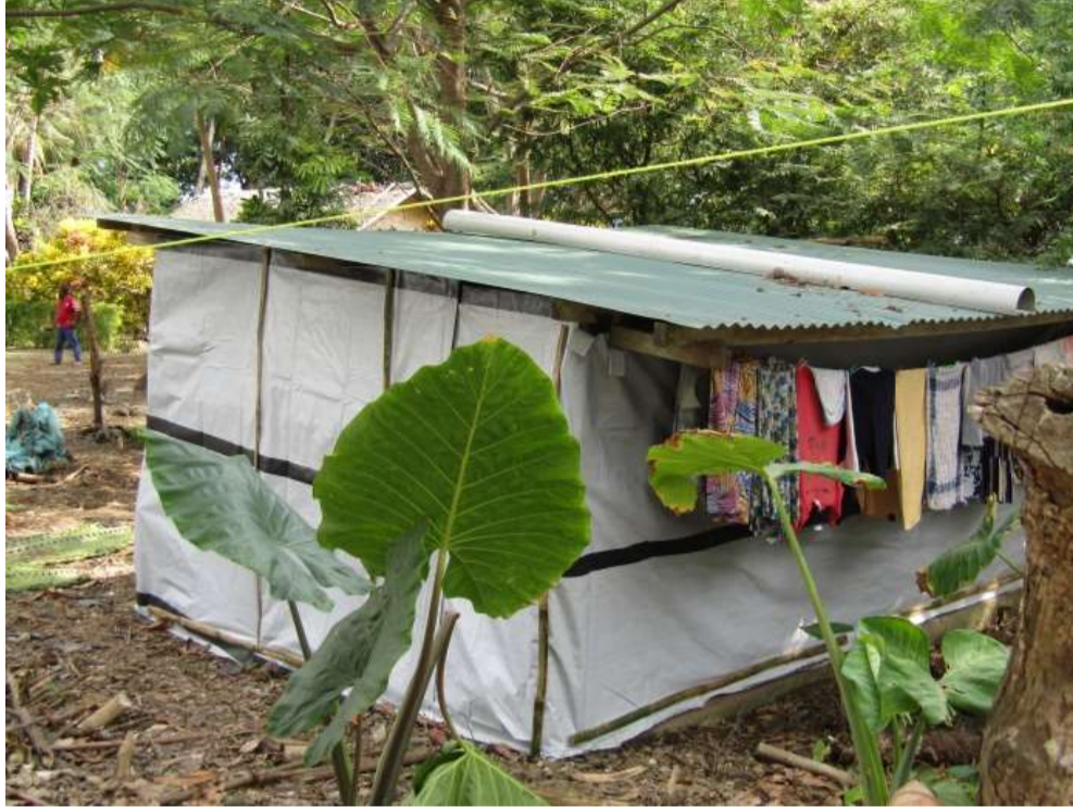
One HH from South Ambae used Iron roof and used Tarps for walling.
