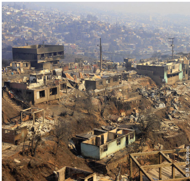
The damage caused by fires in the ravines of Valparaíso is often extensive. Entire neighbourhoods were burnt down by the fire in April 2014. The same areas were again affected by a fire in January 2017.
