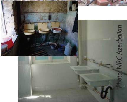
Bathrooms before and after upgrade
