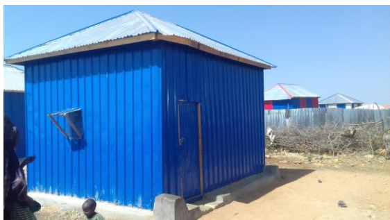
Transitional shelters for Returnees in Baidoa – Intersos
