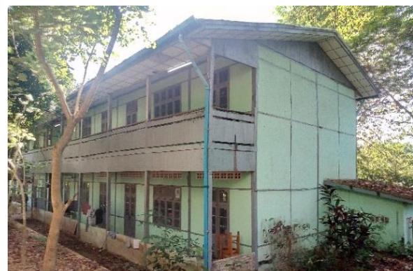
Figure 65: No sign of any distress
