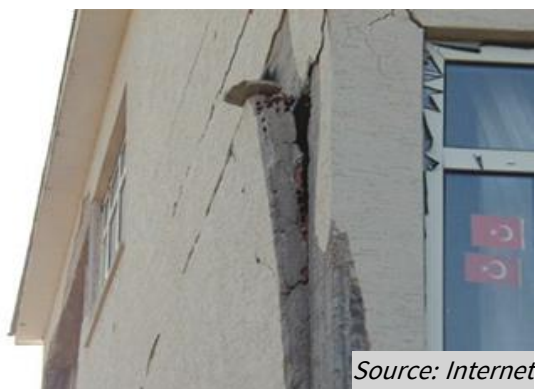
Figure 84: Columns out of plumb or storey leaning
