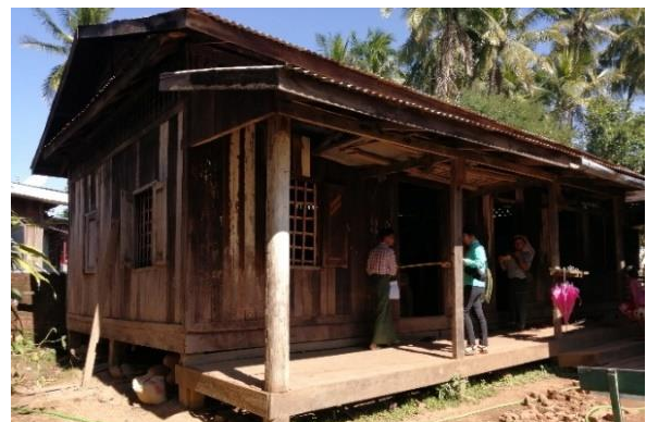
Figure 60: No sign of any distress (Timber building)
