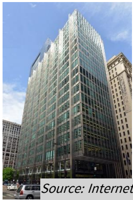
Figure 79: No sign of any distress
