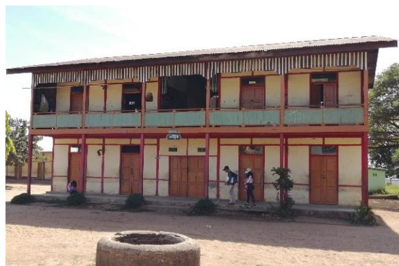
Figure 14: Brick Nogging building
