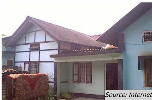
Figure 64: No sign of any distress
