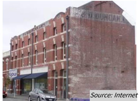
Figure 73: No sign of any distress
