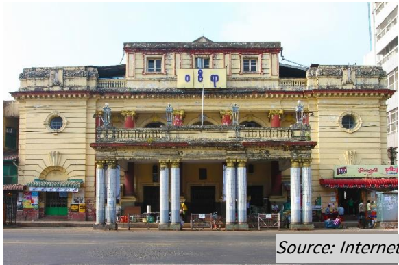
Figure 72: No sign of any distress
