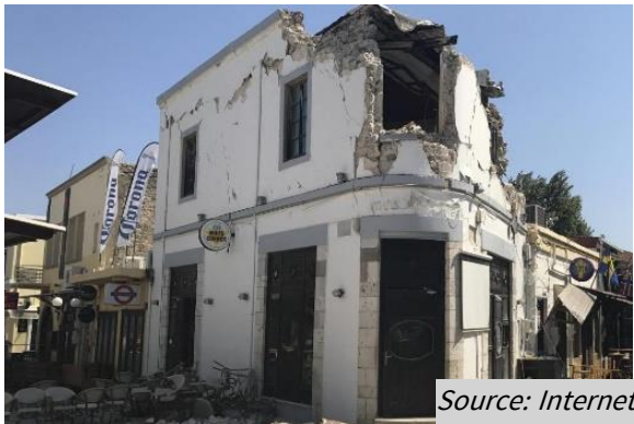
Figure 76: Partial collapse
