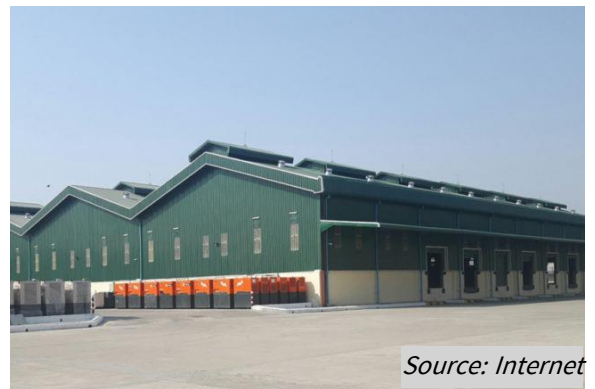
Figure 28: Other occupancy (Warehouse)
