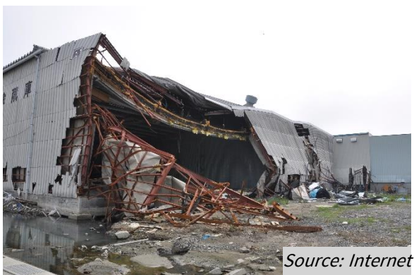
Figure 81: Partial collapse
