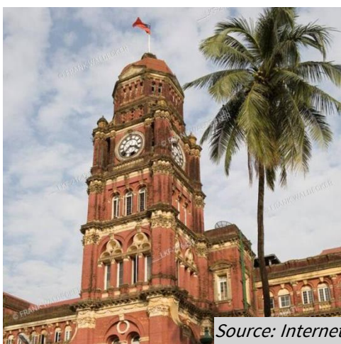
Figure 37: Tower, parapet, chimney
