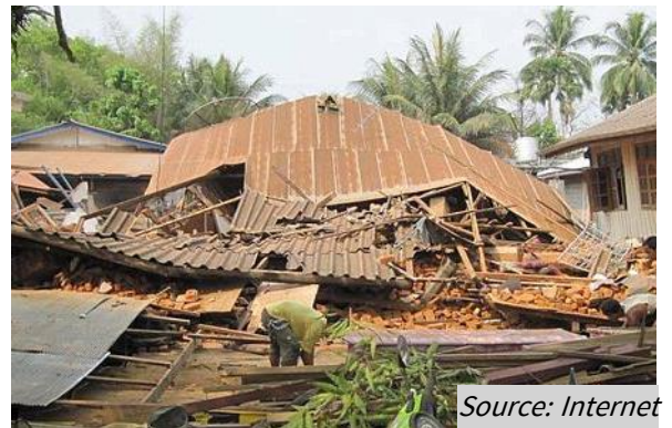
Figure 69: Total collapse
