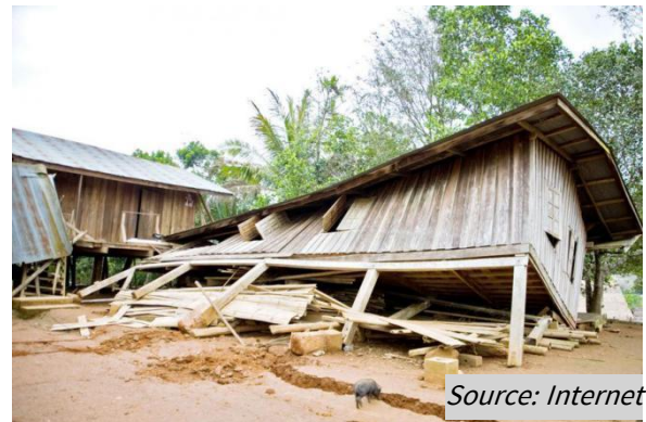
Figure 63: Total collapse
