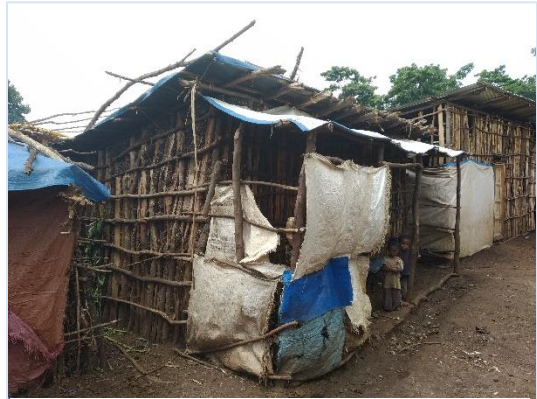
Figure 3 Shelters in Chirico (7) returnee site (Yergachefe) by Shelter
