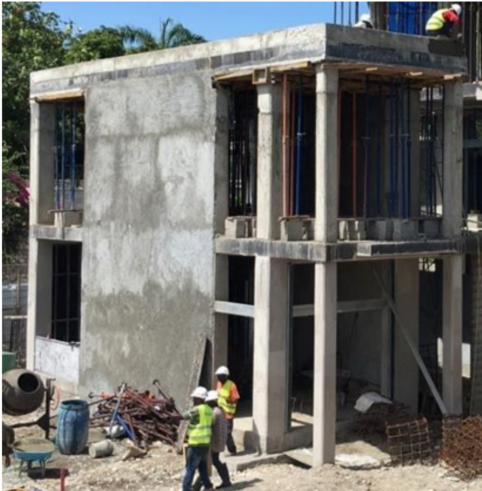
Figure 5: Special reinforced concrete shear wall (unidirectional) in full construction
