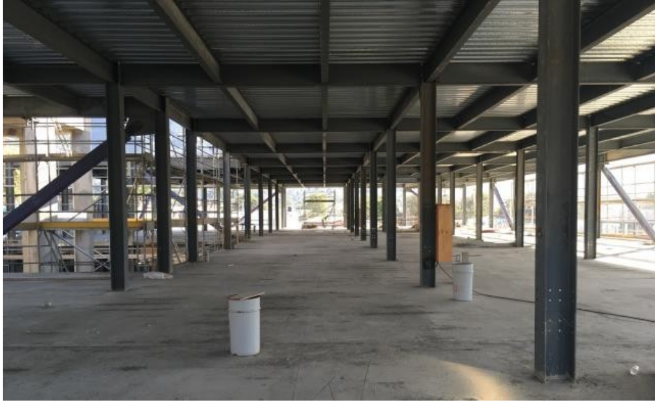
Figure 4: Example of steel structure construction
