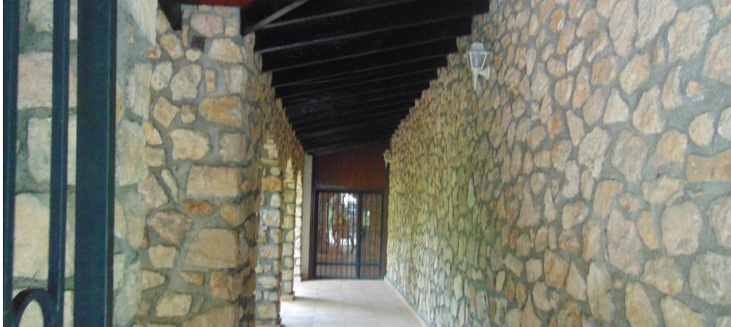
Figure 6: Construction with rock masonry walls
