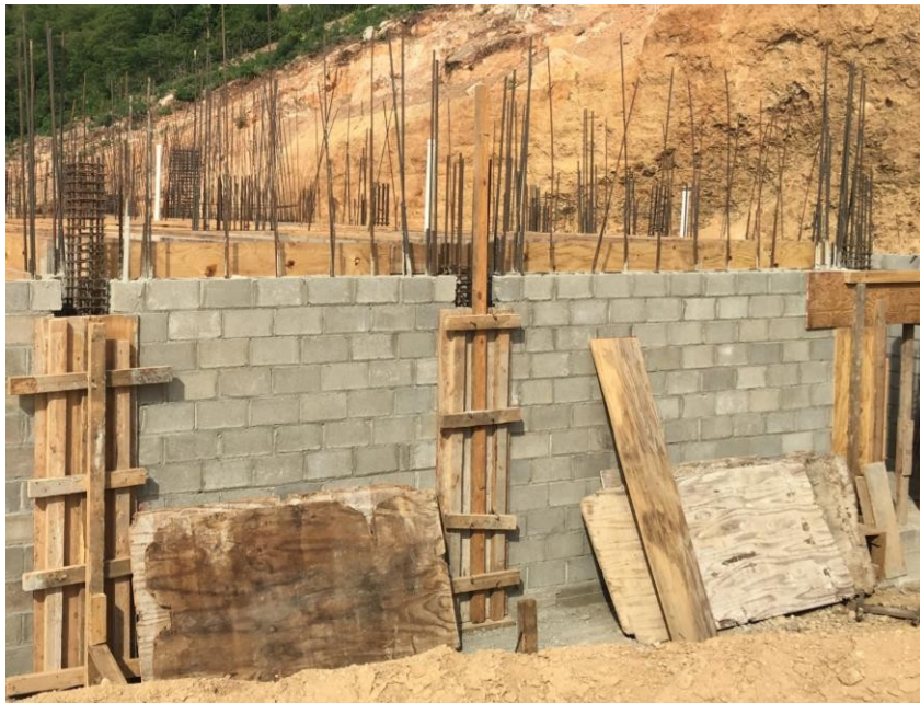
Figure 7: Construction of a concrete block masonry shear wall
