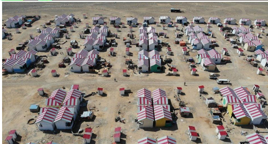
Aerial view the relocation site in Girible settlement
