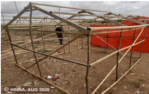
Photo: An emergency shelter under construction in Afgooye.
