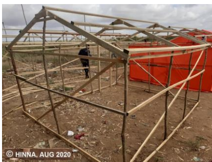
Emergency shelters by HNNA to displaced households in Afgoye
