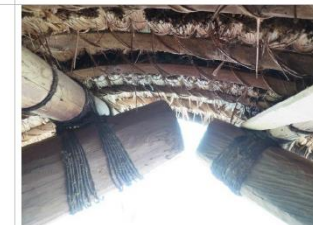
Having separate roofs for veranda and house is a good practice to avoid the whole roof being blown off by strong winds. Aldeia Siscoelema (Liquiçá).
