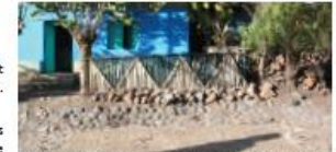
Surface drainage system to prevent from erosion and flooding near Bahir Dar, Amhara. © O. Meles
