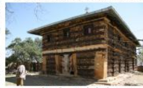
Church with horizontal seismic timber bands or «monkey heads» in Debre Damo monastery in Tigray. CC- Travel Afkonado
