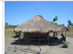
Houses are oriented with the short walls perpendicular to the dominant wind direction, reducing impact on the house. Here the wind comes from the sea, right in the back of the house. Aldeia Kuluhun (Manufah).
