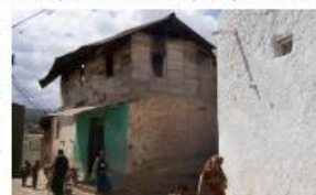
Heavy ground floor and light upper floor in Harar. The upper parts of the walls have a decreased thickness and/or are built with materials lighter and more flexible than those used for the lower parts. CC- IWH
