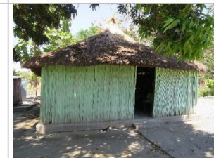
Houses are oriented with the short walls perpendicular to the dominant wind direction, reducing impact on the house. Here the wind comes from the sea, right in the back of the house. Aldeia Kuluhun (Manufah).
