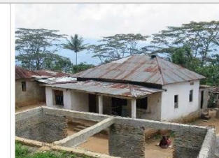
Having separate roofs for veranda and house is a good practice to avoid the whole roof being blown off by strong winds. Aldeia Siscoelema (Liquiçá).
