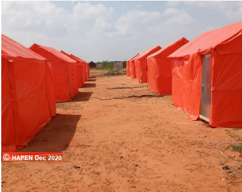
Photo: Emergency Shelters constructed by HAPEN for new IDPs in Dollow
