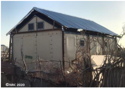
© NRC 2020 An upgraded RHU constructed by NRC by UNHCR funds in Barbera
