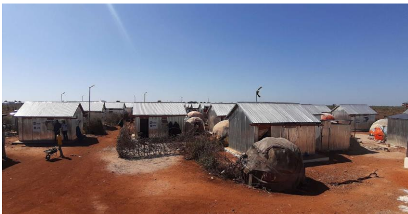
Photo: Transitional shelters constructed by ACTED in Baidoa between September and December 2020.
