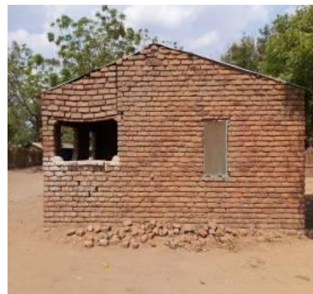
Walls with insufficient thickness and an important height are dangerous in the events of a disaster as they are not stable enough. CC - Ignasio Ngoma
