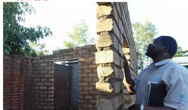
Walls with insufficient thickness and an important height are dangerous in the events of a disaster as they are not stable enough. CC - Ignasio Ngoma
