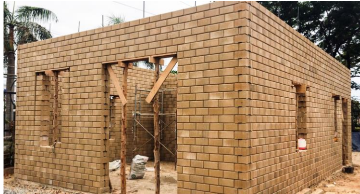
Interlocking Compressed Stabilized Earth/Soil Brick
