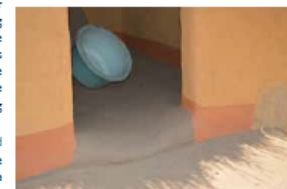
Well maintained earth floor in Chitungulu, Nkhata Bay. © Jon Twingi.
