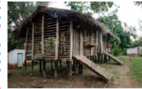
Raised constructions help protect small animals like goats or chicken from floods. These constructions are very common throughout the country. This is an example of raised goat pen at Nainingazi Farm Training Centre. © Gernischaw C.
