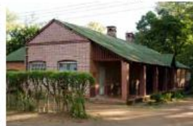
British colonialism also introduced in Malawi the use of fired red bricks, regular and paced windows and doors, concrete or burnt bricks lintels and roofs covered with corrugated iron sheets Mission in building in Blantyre. CC: Camichaw C.
