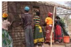
Images of the construction process. © Jamie Richardson (CRS)
