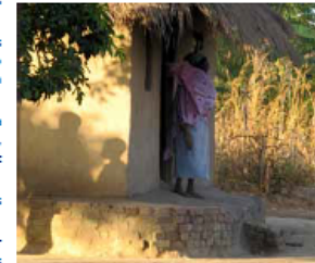
Some families protect the ends of the raised earthen mound with fired bricks or stones. House in Mtetere. © Jon Twigg
