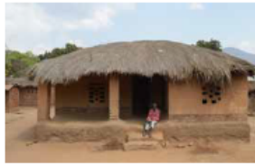
Houses constructed using adobe bricks, render and earth mortar like this one (Chisoka, Rumphi District) responded well to the important floods in 2015 (CRS, 2020) as the design developed over centuries provides protection from the elements. Other than some minor repairs, some of these houses were in good condition and allowed the families to return to their homes once the floods had subsided. © Jon Twigg
