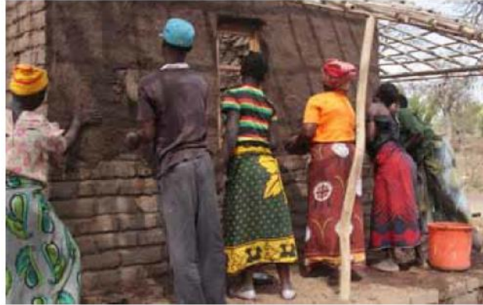
Rendering a house in a training by CRS. © CRS
