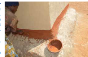
Women applying a red earth based painting in Chisi, Nzimba. © Jon Twingi.
