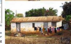
These two houses would be semi-permanent according to different authors as they are built with a mix of materials. The one on top has burnt bricks and thatched roof (Kachopetsonga, Nkhata Bay- © Jon Twigg). The other one has adobe brick walls and metallic roof (Lilongwe- © Urbanopolita)
