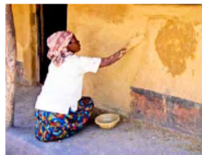
Women cladding a wall with earth plaster. © Gregory S.
