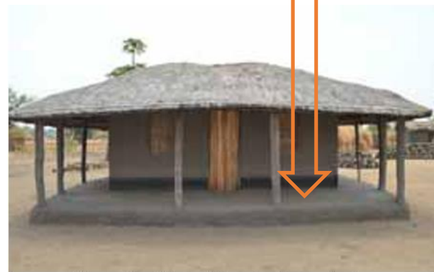
Verandas ( khonde ) and other exterior covered spaces where many daily life activities take place as these shadowed spaces are very comfortable in hot days. House in Penganga, Ntcheu. © Jon Twingi
