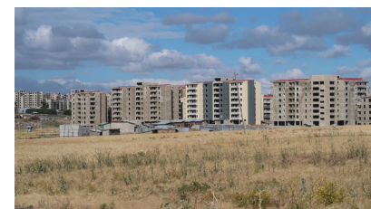
Condominiums under construction in Addis Ababa. © v. M
