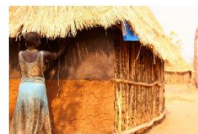
Active participation of beneficiaries through mud plastering and thatching. © Mikea Mohammed - IOM
