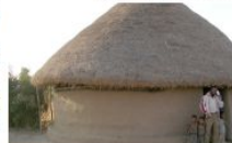
Ventilation is made possible thanks to the absence of plaster in the upper part of the walls in the Alaba Houses. (SNNPR). © Laurence Fontana
