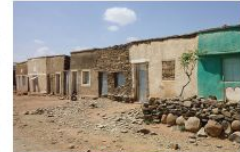
Houses with stone masonry walls in Tigray. © Bernard Diagne
