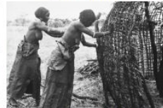
Construction of a Borana 'bird's nest' house. CC-National Museum of World Cultures
