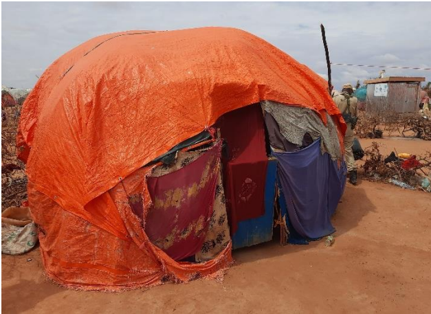
Tarpaulin plastic sheet reused in a buul (Doolow) (CC – Enrique Sevillano Gutiérrez – CRAterre)
