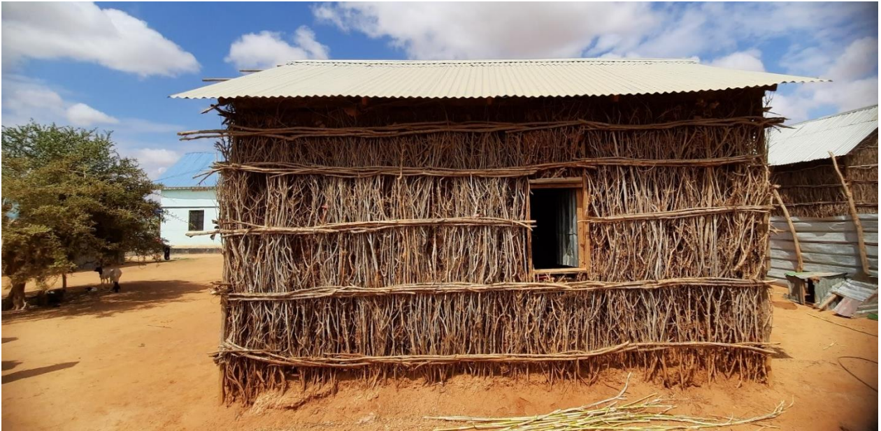
Use of local lumber and branches of small sections for the structure of a baraako house without plaster (CC - Enrique Sevillano Gutiérrez - CRAterre)
