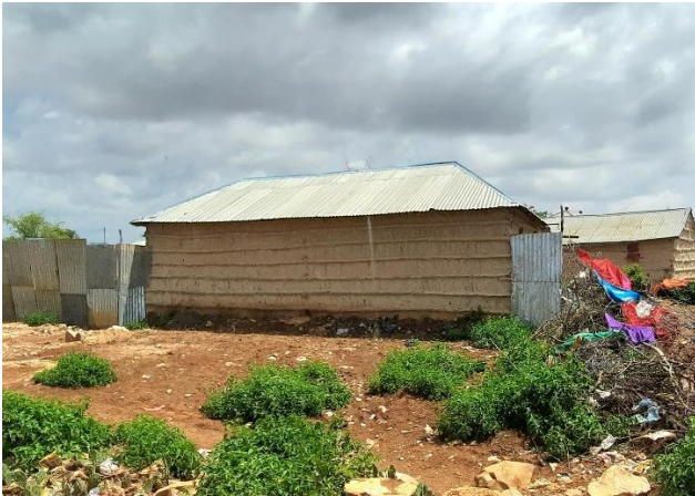
CGI sheets roofs are more and more prevalent in sedentary constructions (Baidoa) (CC – Enrique Sevillano Gutiérrez – CRAterre)
