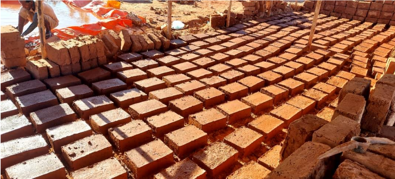
Adobe blocks production (raw earth + water + sand) in Doolow (© IOM)
