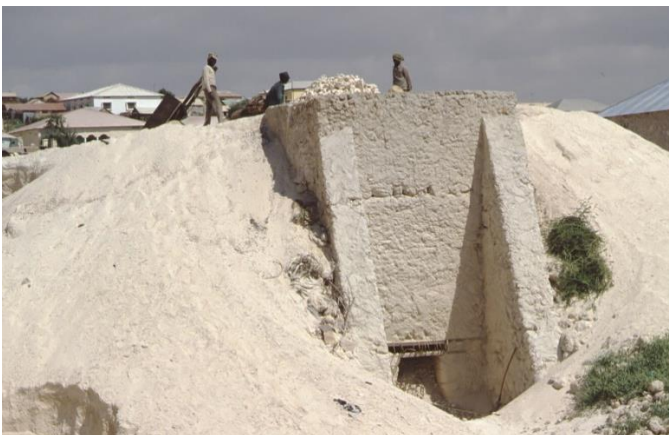
Kiln for lime production using coral limestone in Merca (South West State) (1980s) (© Thierry Joffroy - CRAterre)
