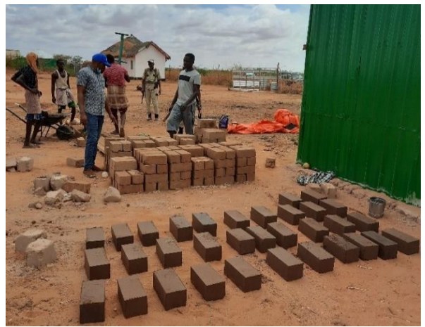
Compressed Earth Blocks production in Doolow (Jubaland) (CC – Enrique Sevillano Gutiérrez - CRAterre)
