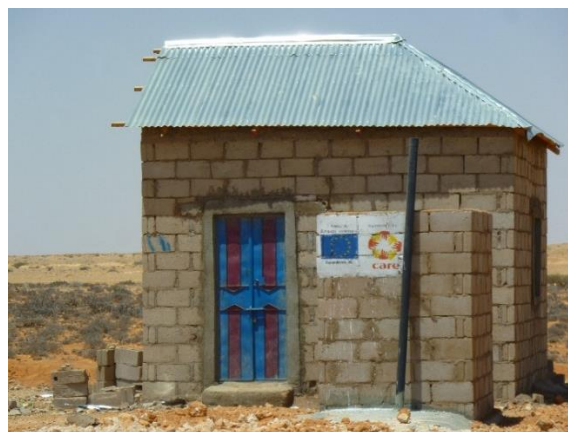
Shelter built with cement blocks with possibility of extension in Garowe, Puntland (CC – Malini Morzaria / EU ECHO)
