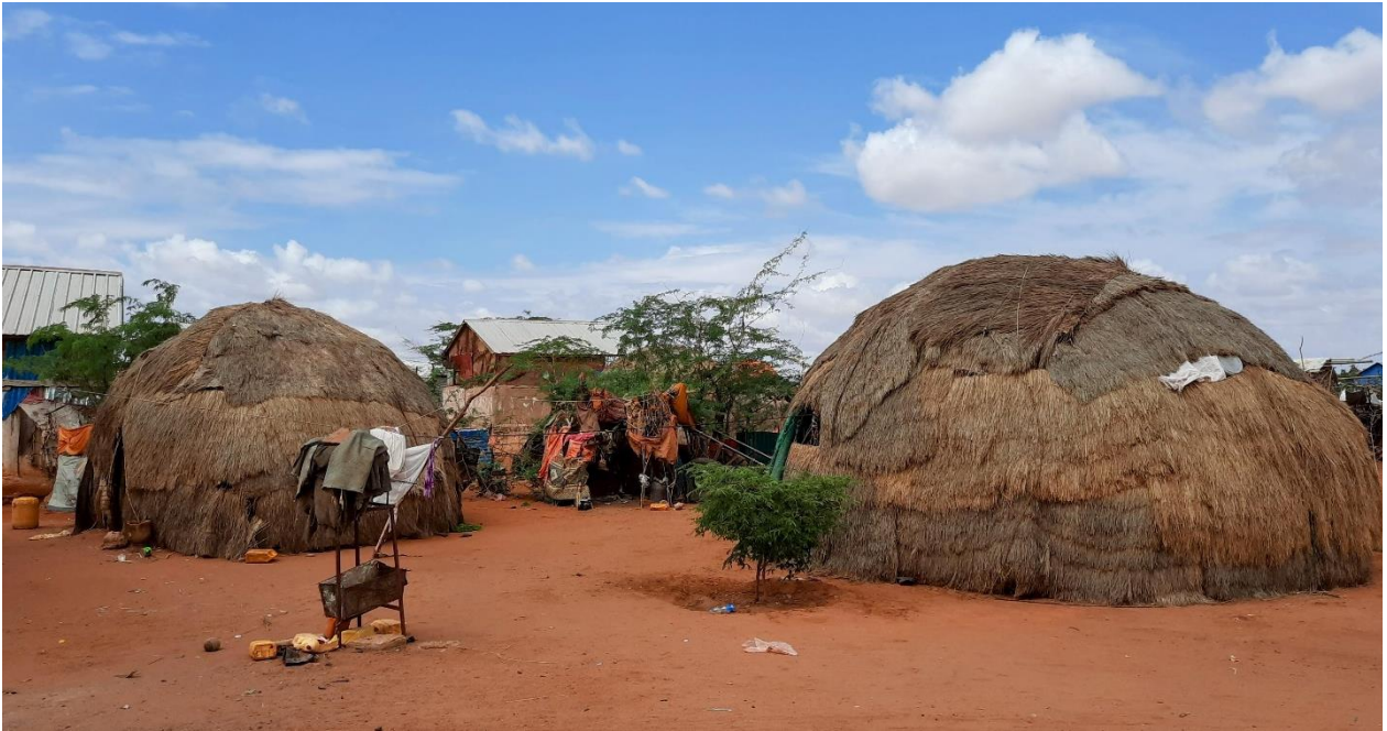
Nomadic constructions ( aqal ) made mostly from plant fibers in Doolow (CC - Enrique Sevillano Gutiérrez - CRAterre)
