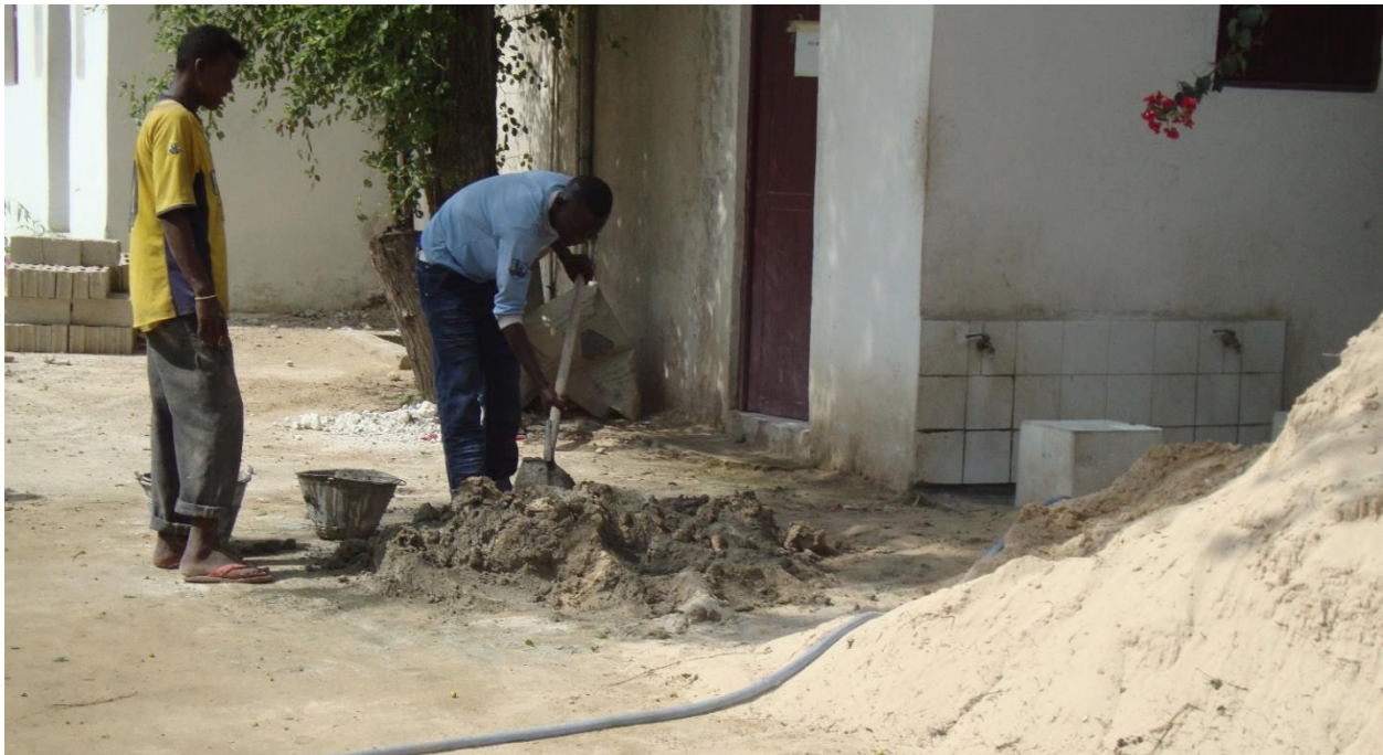
Use of sand for cement mortar production CC – Cospe
