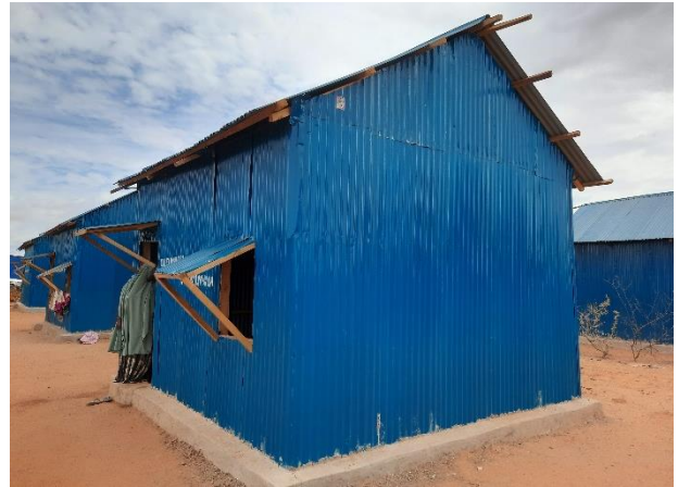
House completely covered with CGI sheets (Doolow, Jubaland) (CC – Enrique Sevillano Gutiérrez – CRAterre)
