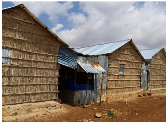
Stone used in foundation and plinths in Baidoa (CC - Enrique Sevillano Gutiérrez - CRAterre)
