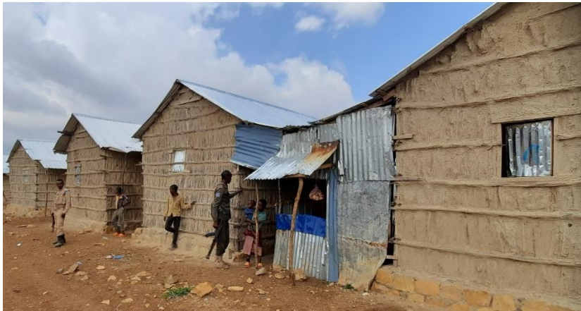
Solution of shelters where each material finds its place in the right part of the building (stone and cement in the foundation and base, wattle and daub in the walls, CGI sheets in the roof), adding value and durability to it. CC – Enrique Sevillano Gutiérrez – CRAterre
