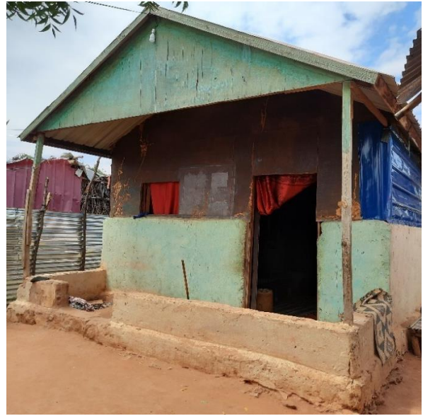
Plywood panels and sawn timber sections used in a shelter in Doolow (Jubaland) (CC - Enrique Sevillano Gutiérrez - CRAterre)
