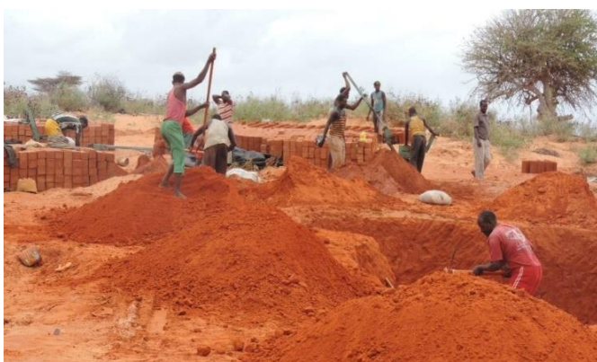
Production of CSEB (Compressed Stabilized Earth Blocks) in Kismaayo (Jubaland) (© IOM)
