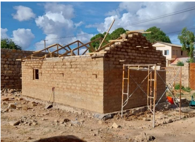
Adobe house (transitional shelter) under construction in Baidoa (© Héctor Esteban – CRAterre)
