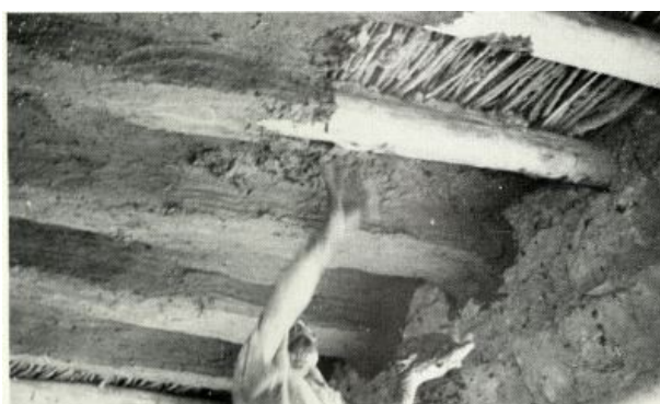
Ceiling with earth plaster – ©Fernado Varanda
