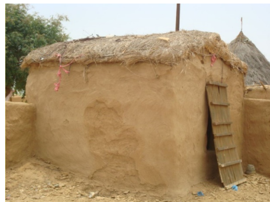
Transitional shelter: earth Blocks, Sa'ada and Harad © CCM
