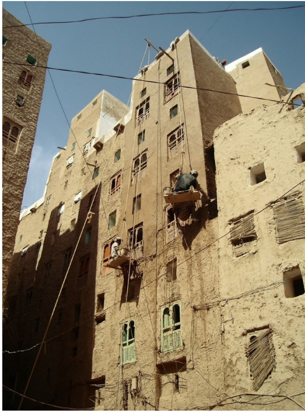
Shibam, maintenance of an earthen tower house © Tom Leiermann
