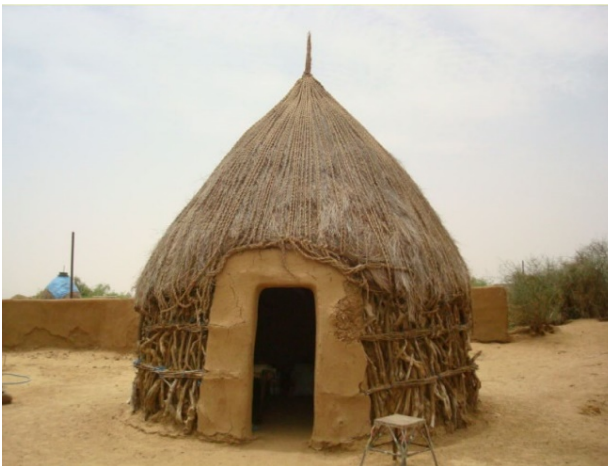
Transitional shelter: Wattle and daub, Harad, Coastal Region © CCM
