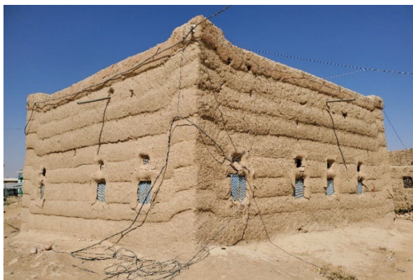
Cob walls, Al-Jawf Gov, Almttoon district, 2021 © YFCA
