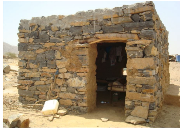
Transitional shelter, stone masonry, Sa'ada, and Amran © CCCM
