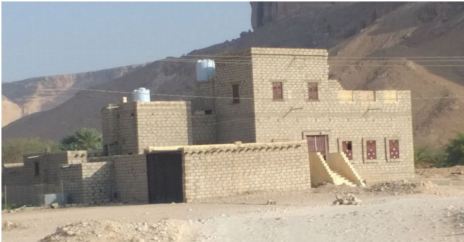
Cement block house Al Hudaidah – ©YFCA
