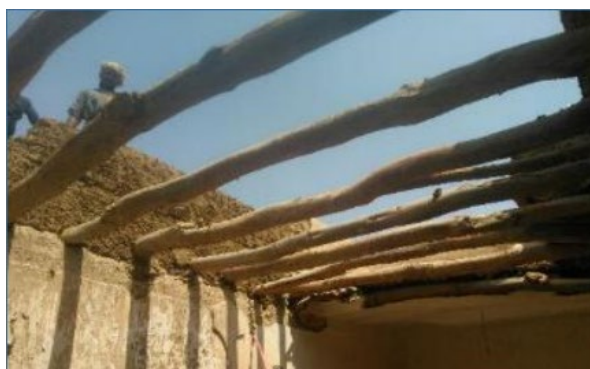
Floor on cob construction – © YFCA
