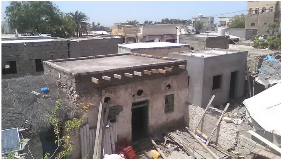
Cement block house Al Hudaidah – ©YFCA
