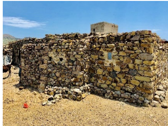
Rubble masonry, Ibb – ©Alezz/ Shelter cluster
