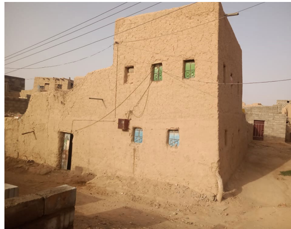
Earth brick building, Shabwa Gov., Almarkha Alsofla Dist., 2022 © YFCA
