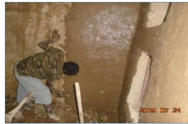
Cob wall mortar preparation and earth plaster © YFCA
