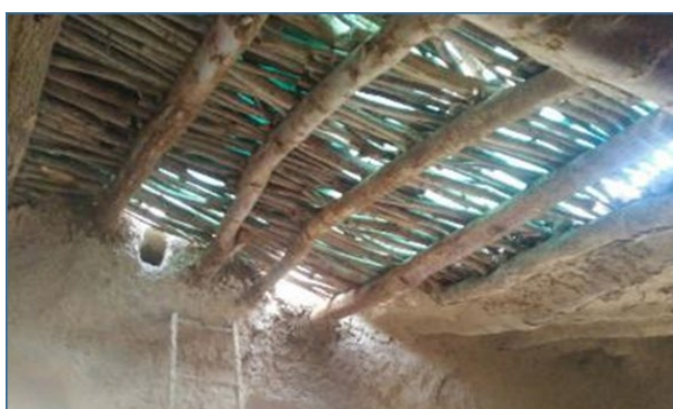
Floor on cob construction – © YFCA
