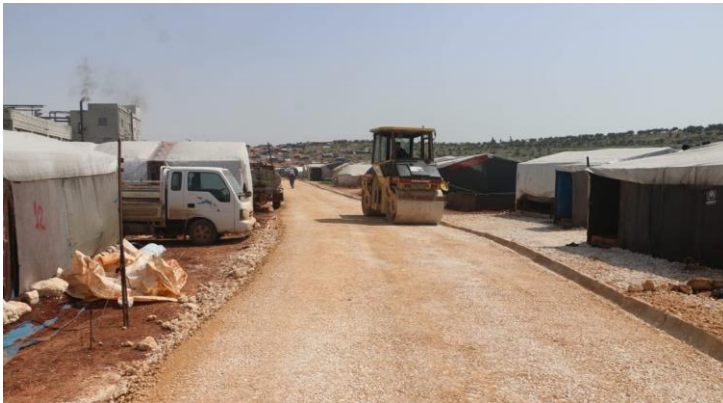
Photo Credit: IYD NW Syria Infrastructure Improvements in IDP sites
