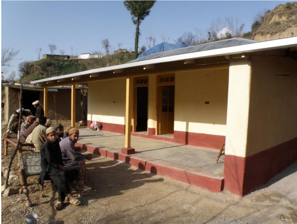
PAKSBAB Straw Bale House - 2009
