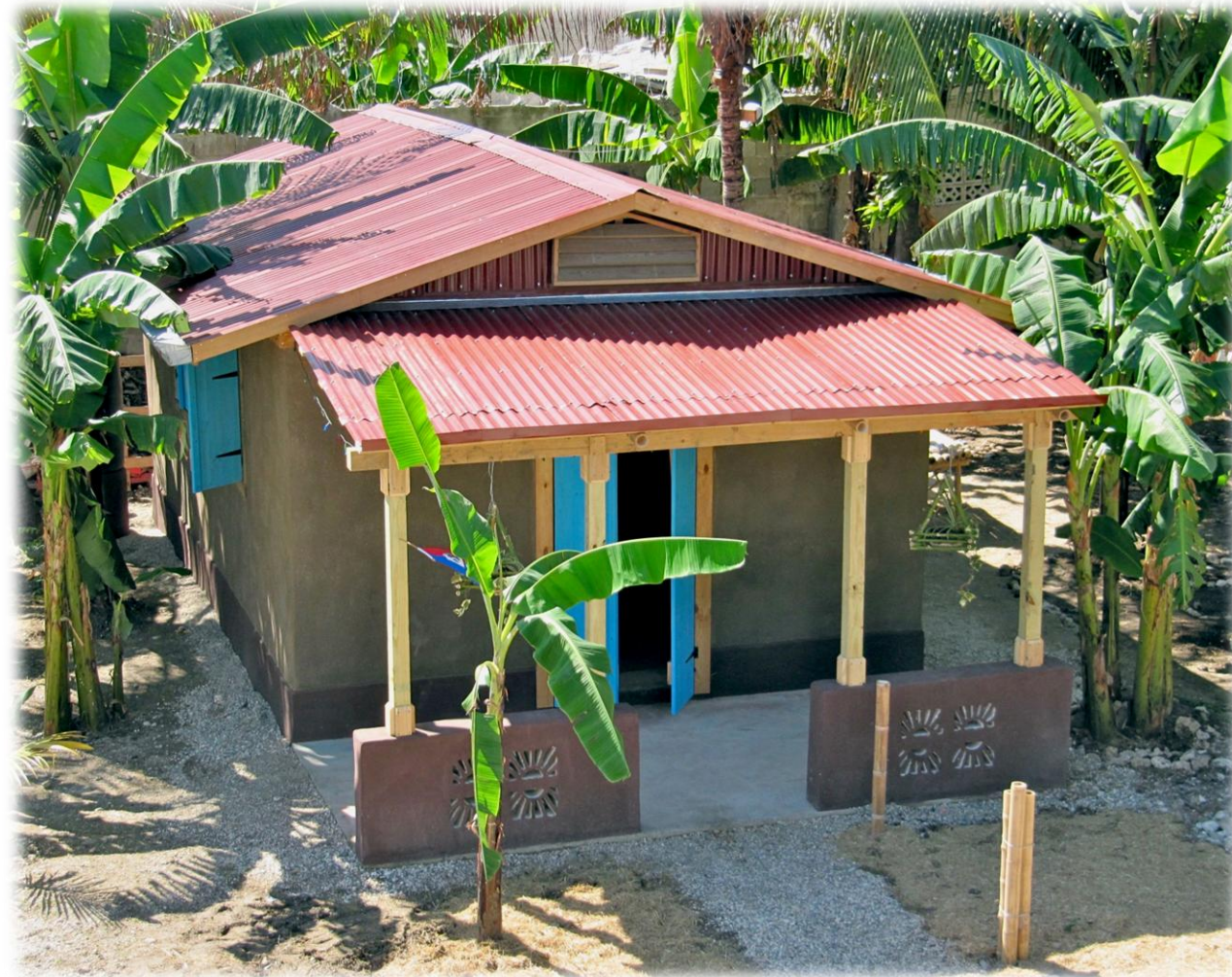
Ti Kay Pay – Small Straw House The First Straw Bale Building in Haiti
