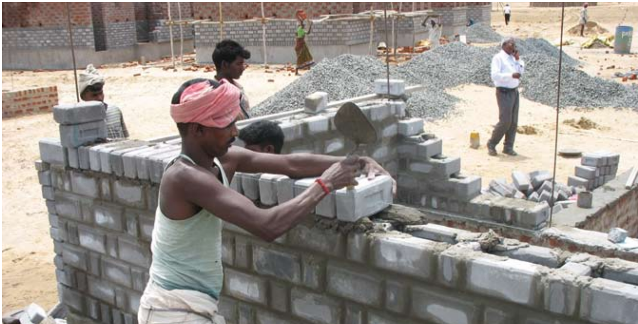
'Rat trap bond' masonry is a cost-effective method, reducing consumption of bricks and mortar.
