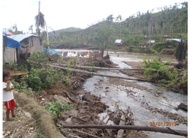
Danger zone in So. Coog, brgy. Mahan-ob. Confluence of Coog creek and Mahan-ob River
