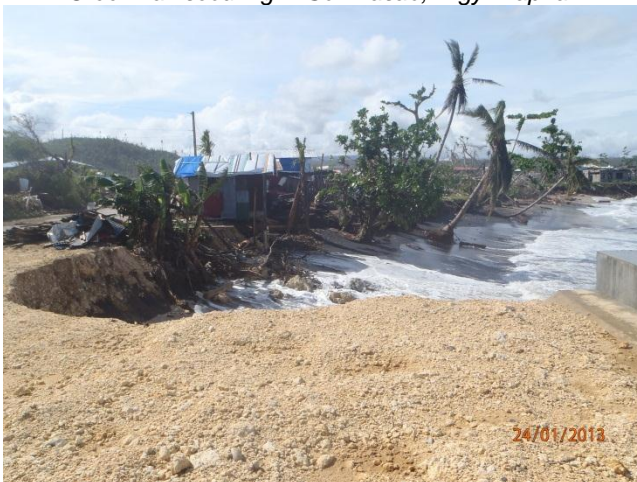
Coastal erosion in Po. Malinawon, Brgy. Central
