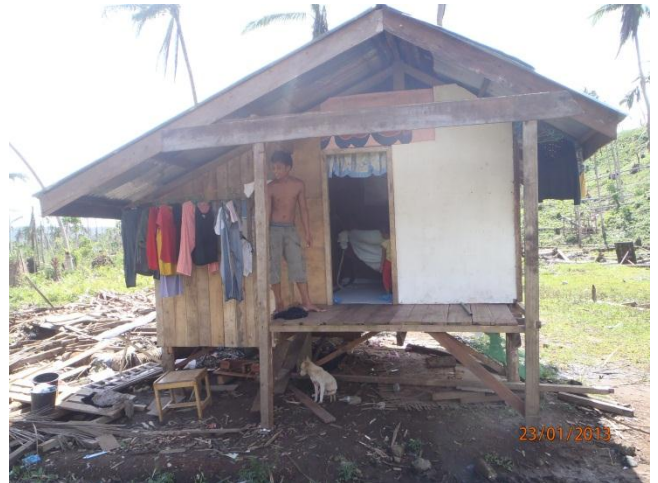
Flood-adaptive houses in So. Abuyuan
