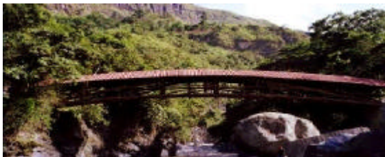
Covered bridge from Jörg Stamm
