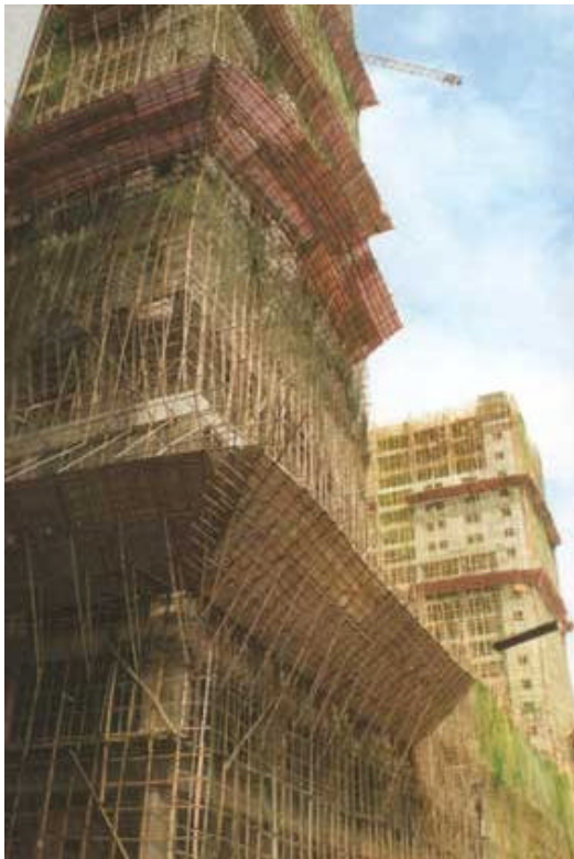
Bamboo canes used for scaffoldings
