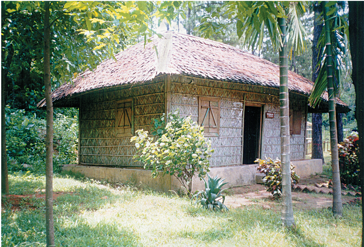
Hut built by BFRI at Chittagong - A pilot project using treated bamboo, wood, Sun-Grass etc.
