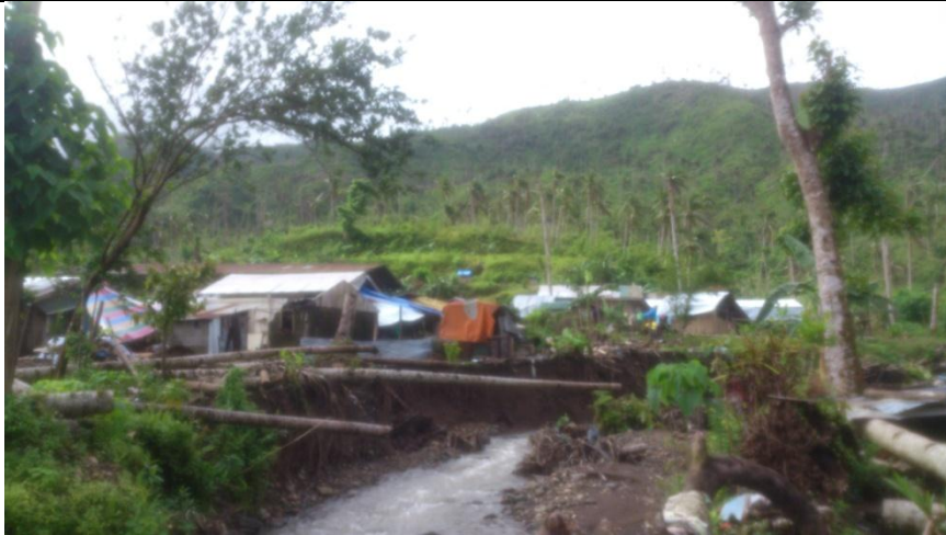
Accelerated river bank erosion in Po. Ipil-ipil, Brgy. Cabasagan
