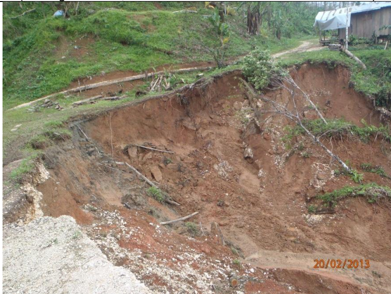
Earth flow in So. 5m along the barangay road (Looking southwest; GPS location: 7°55'54.464"N 126°18'9.746"E)
