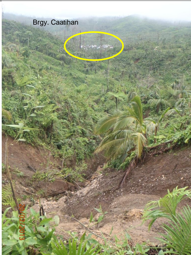
Earth flow noted along the barangay road to Brgy. Simulao. (Looking northeast; GPS Location: 7°53'18.824"N and 126°16'45.12"E )
