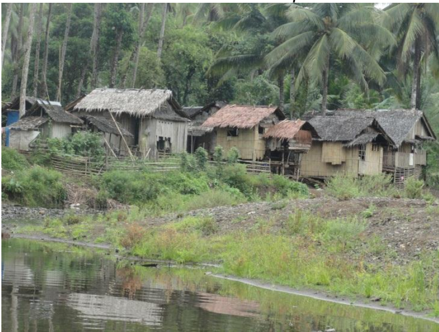
Houses at risk in Phase 2 Brgy. Mainit
