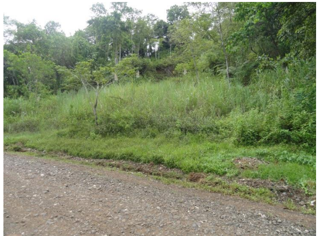
Reactivated rotational landslide directed toward Mainit Brgy Hall and Day Care Center
