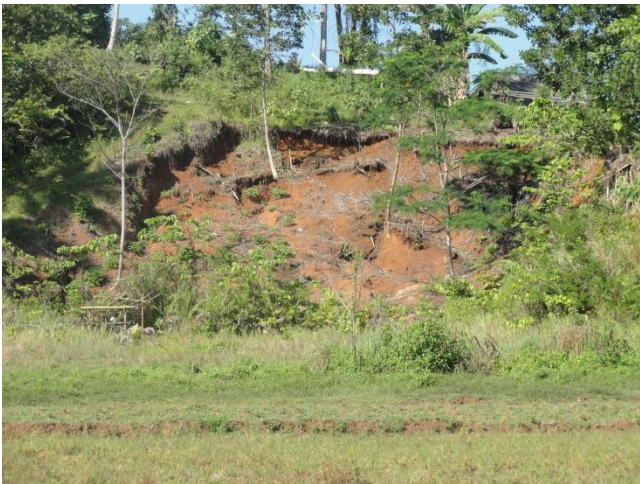
Active slope failure along the road from So. Mangga to So. Magong-ong
