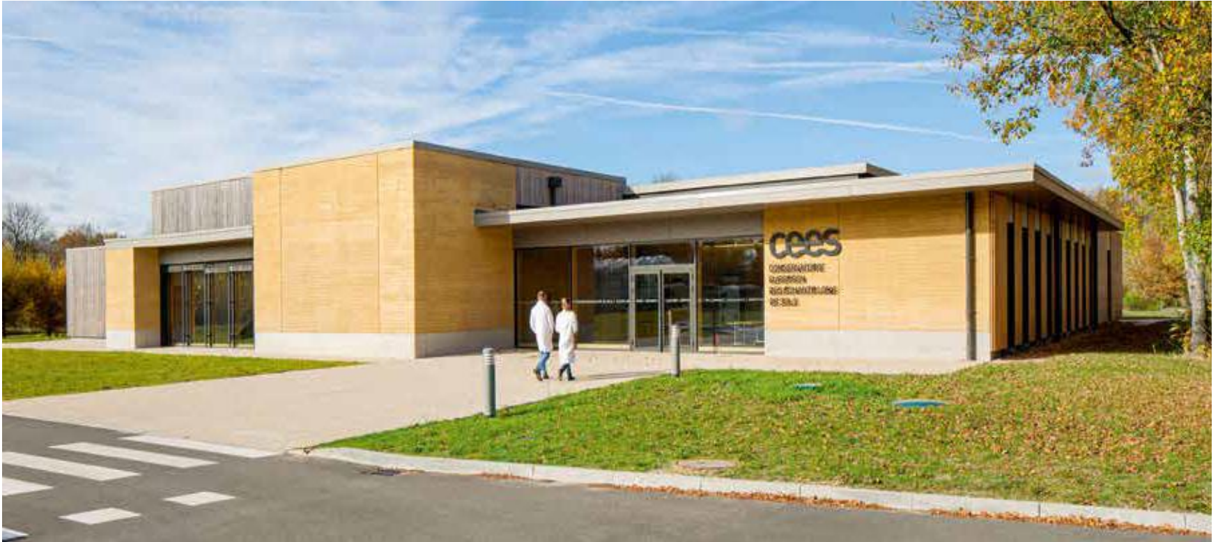
France, National Institute for Agricultural Research (INRA) on the university campus in Orléans, France Nama Architects
