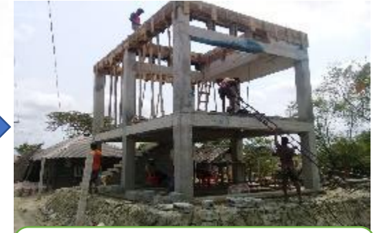
All Frame & Structures works
