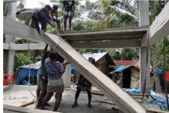
Block, Ferro-Cement Channel and Stair Installed in Building
