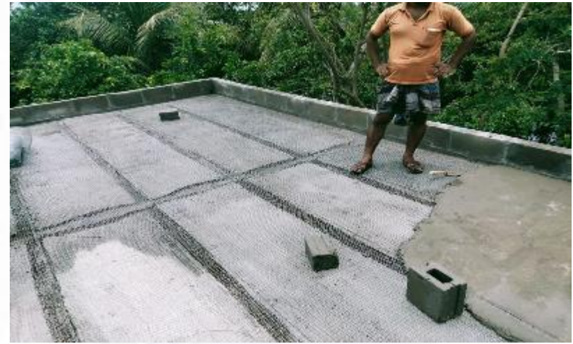
Ferro-cement Channel Manufacturing
