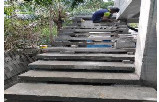
Block, Ferro-Cement Channel and Stair Installed in Building
