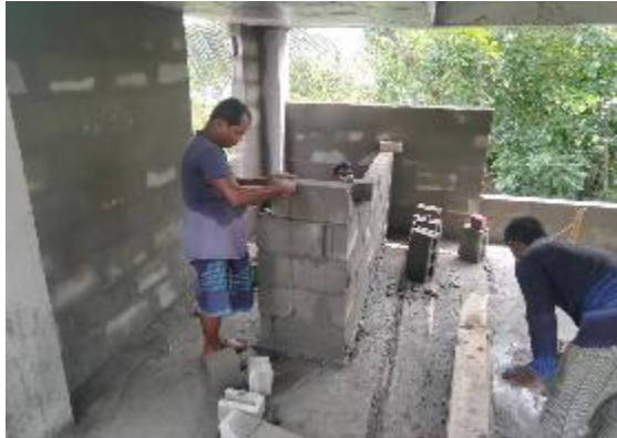
Block, Ferro-Cement Channel and Stair Installed in Building
