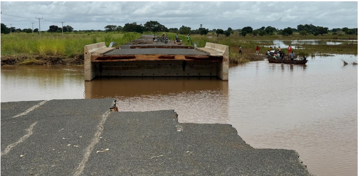
Figure 1. Interruption of National Road N281, the main access route to Buzi district headquarters.
