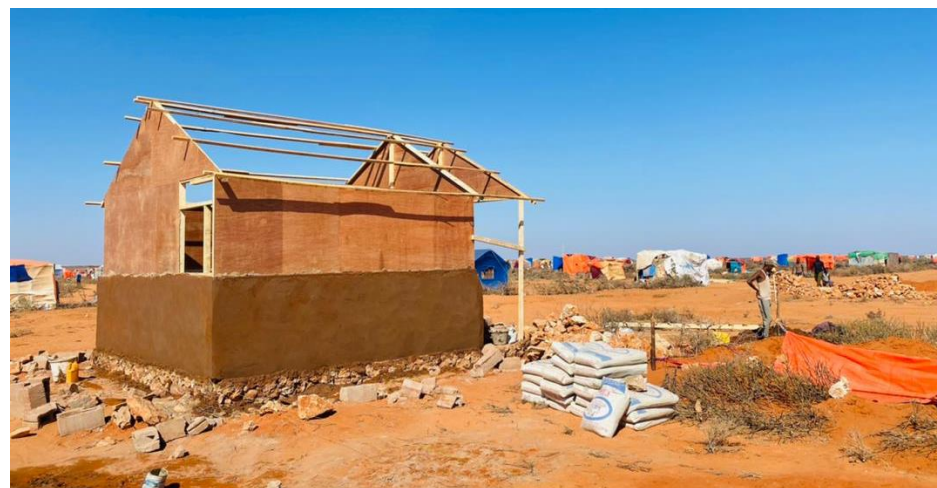
Construction of hybrid shelters in Kismayo - UNHCR/NRC
