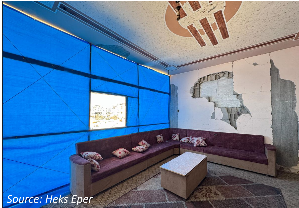
Sealing off kit used to create a temporary wall
