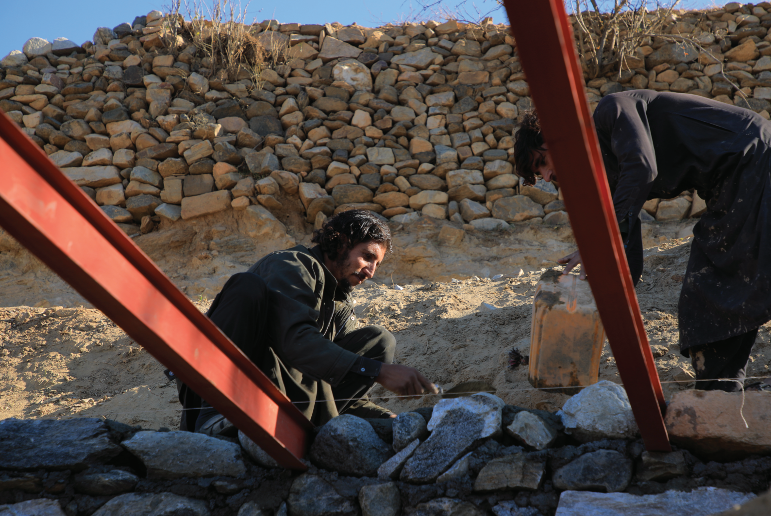
Shelter Construction, Khost, Afghanistan. © UNHCR
