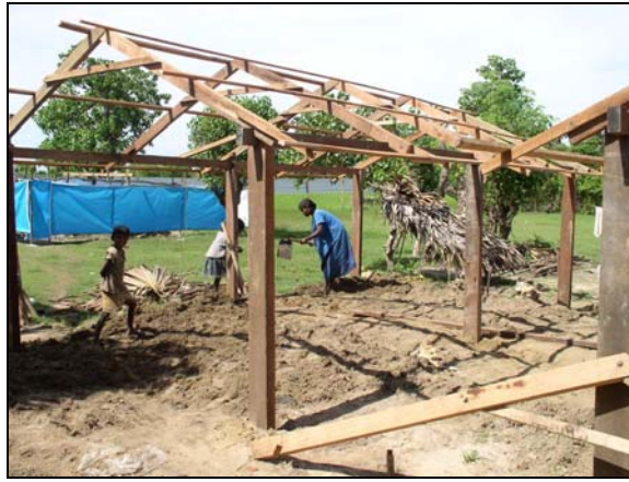
Details of roof Timber structure (Source: JSAC)
