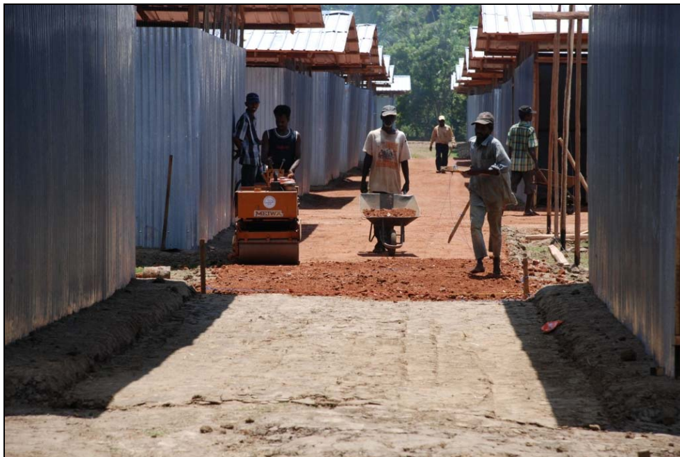
Corrugated Tin Gable Roof; Corrugated Tin Walls
