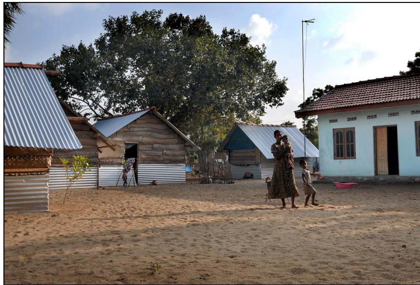
Corrugated Tin Sheet Gable Roof+ Cadjan nd Corrugated Tin Sheet Walls (NRC photos by: Sujeewa de Silva)
