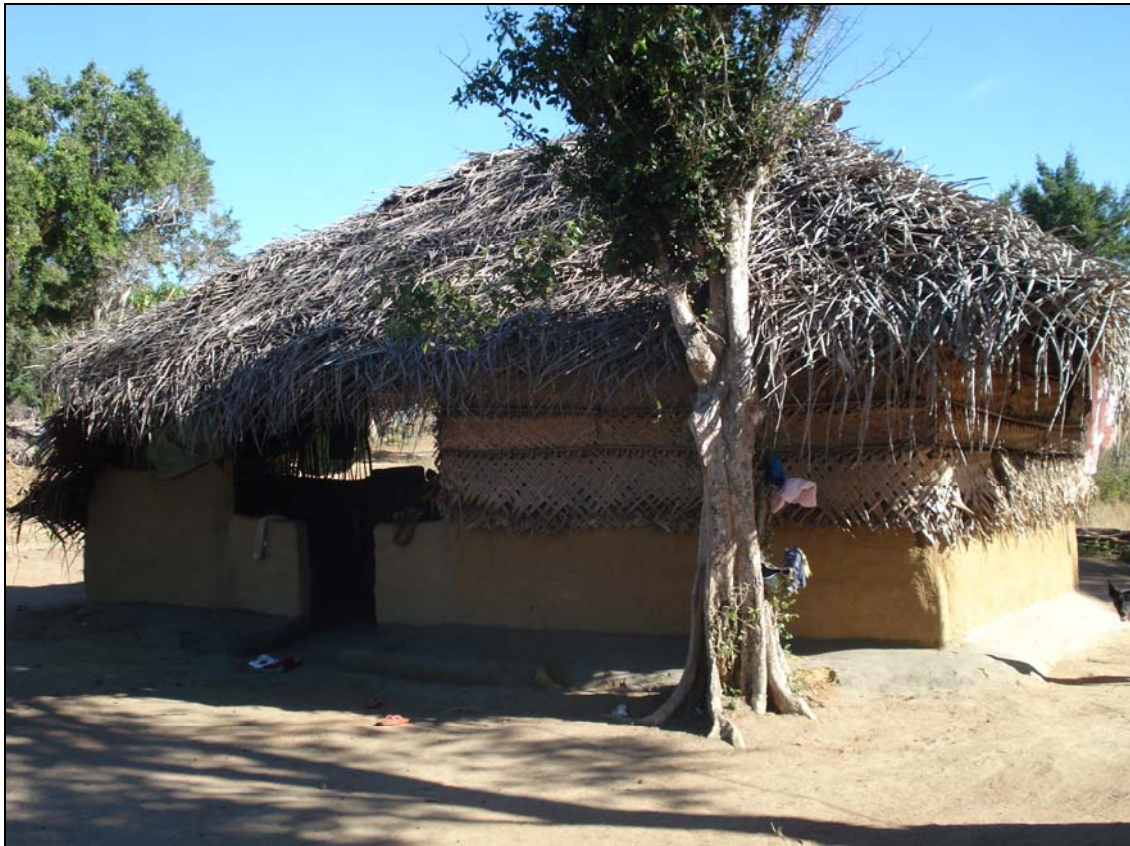
Cadjan Gable Roof; Mud & Cadjan Walls
