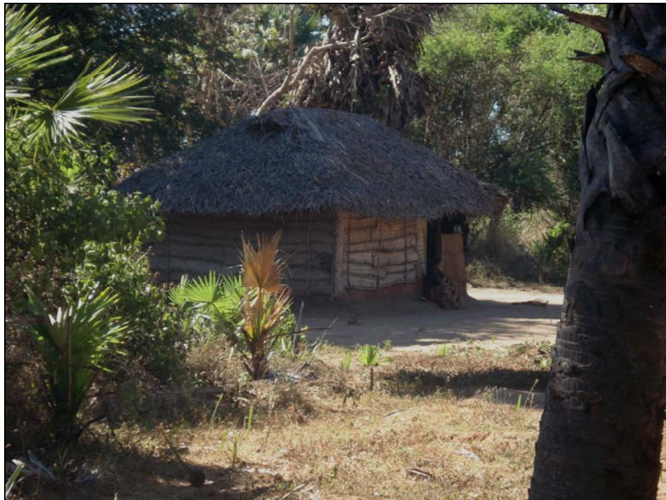
Cadjan Hip Roof & Cadjan Walls
