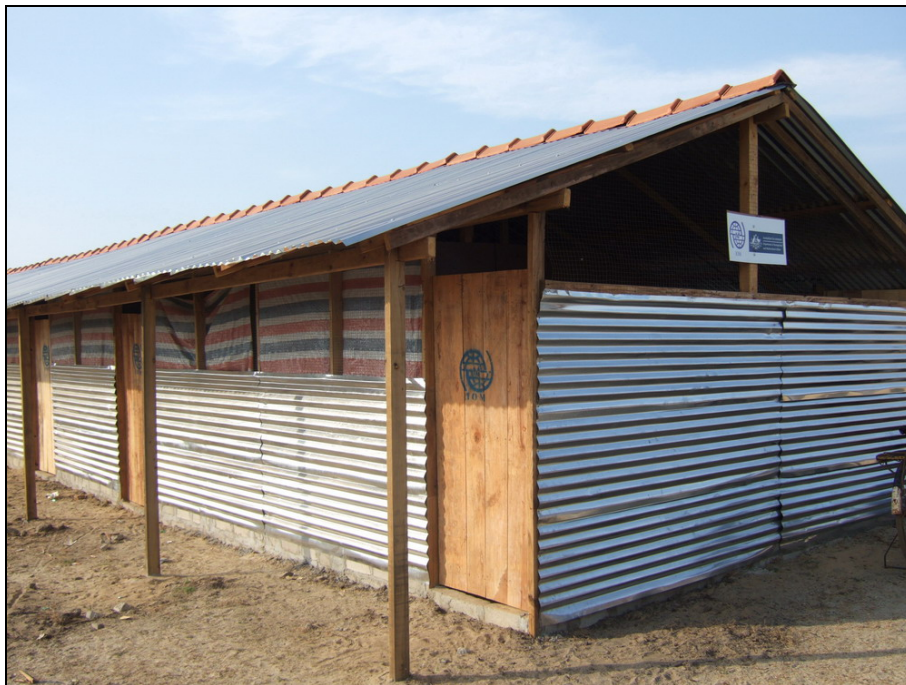
Corrugated Tin Gable Roof; Corrugated Tin + Plywood Walls
