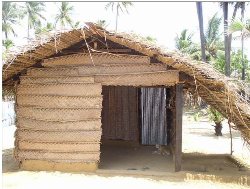
Cadjan Gable Roof ; Cadjan Walls
