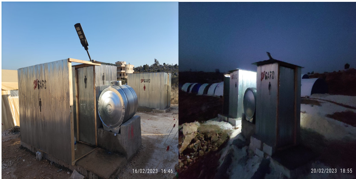
Latrine installation in Termanin
