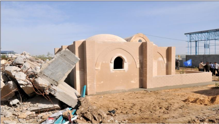
UNRWA, Compressed Earth Block (CEB) shelters, are not the permanent solution, but they are one transitional option for those who are still living under tents or in damaged houses.
