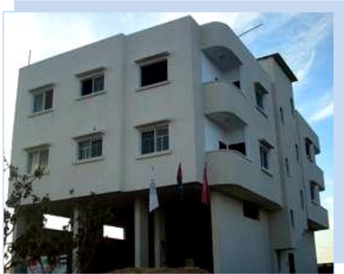
4 apartment building reconstructed in Jabalia
