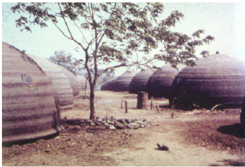
An example of pre-fabricated housing.
