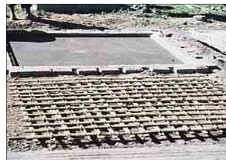
Fig 11.10: Bamboo reinforcement
