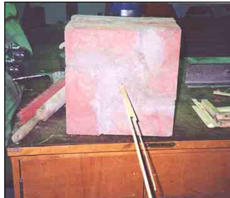
Fig 14.11: Brick with embedded splint
