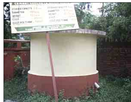
Fig 11.9: Bamboo-reinforced concrete silo
