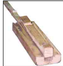
Fig 14.4: Epoxy glued support end
