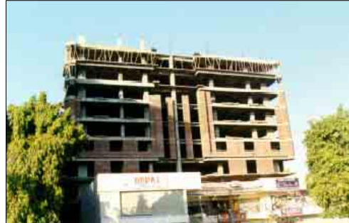
Fig 4.10: View of a typical RC complex
