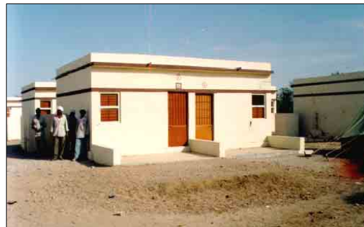
Fig 4.6: Typical cement block masonry house
