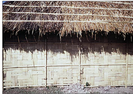
Fig 11.4: Bamboo mat wall
