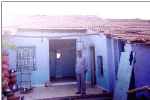
Fig 4.5: Typical brick masonry house
