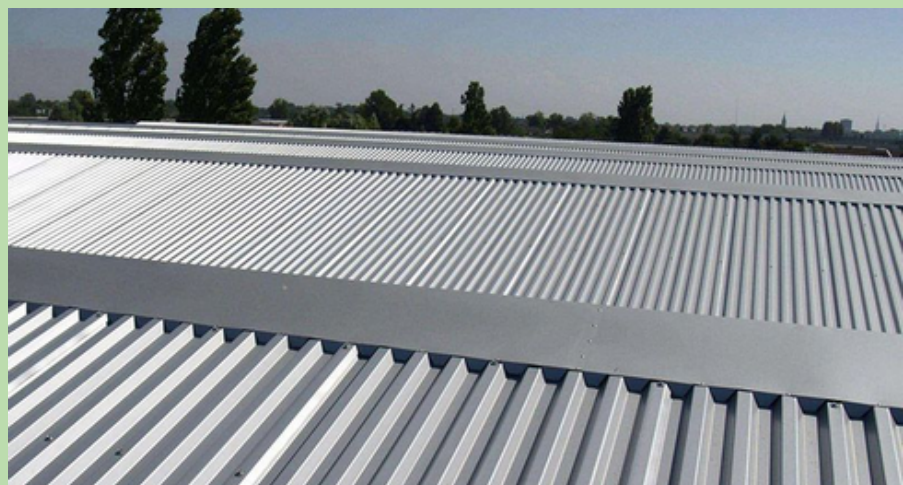
Galvanized Steel Roofing
