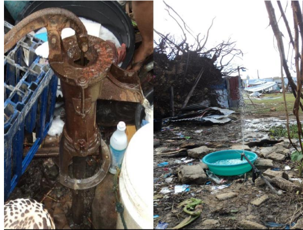
Figure 13: Level I and III water supply systems in poor sanitary conditions increase public health risk
