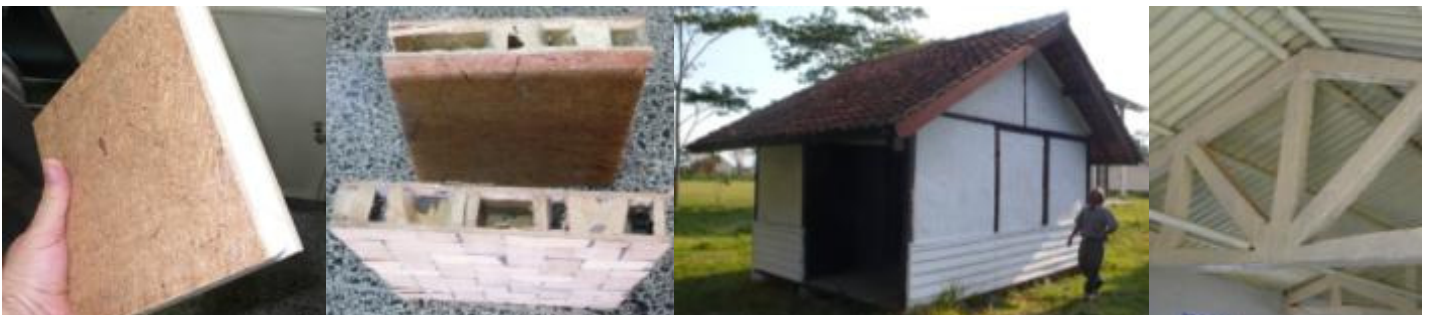
DETAIL 1 2 3: DPU BUNDUNG RESEARCH CENTER- BAMBOO FIBRE POLYSTYRENE COMPOSITE PANEL, HOLLOW CORE BAMBOO PANEL, BAMBOO PLASTER HOUSE DETAIL 4: BAMBOO RESIN COMPOSITE TRUSS, INDIA
