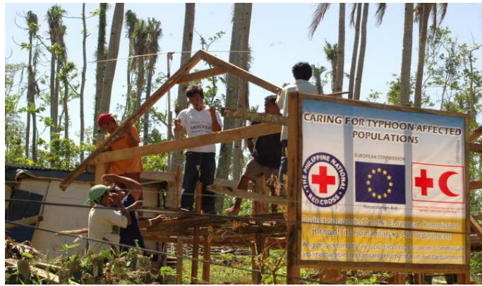
Community members building homes in the spirit of bayanihan.
