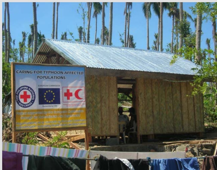
A model home constructed in Albay.
